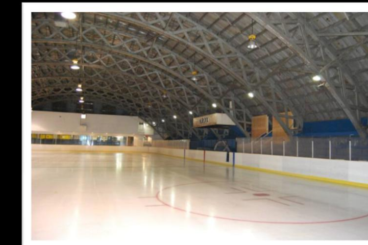
Wood Truss Roof
