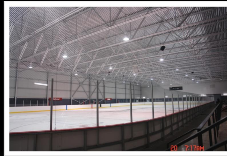
Flat Steel Truss
