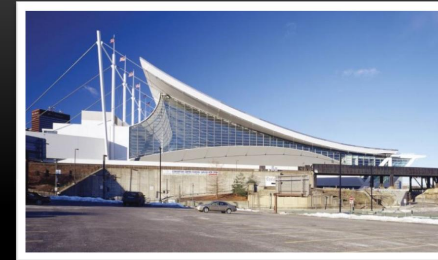
Cable Supported Roof
